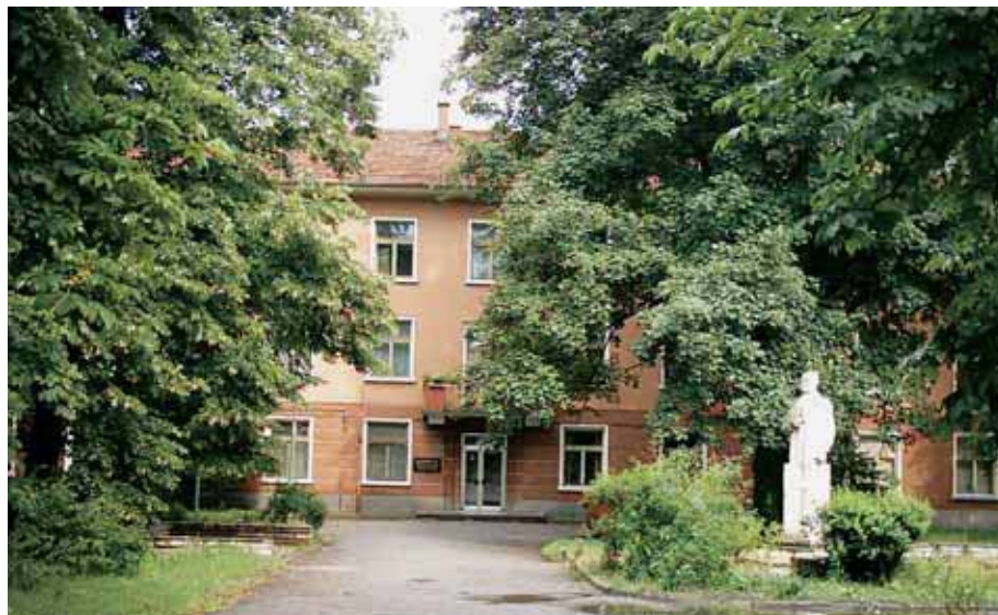
● Maritsa Main Entrance House, built in 1960. It is surrounded by rare and valuable dendro species and comprises mainly administrative and library premises, some labs, and offices of researchers. The other Units are scattered in an Arboretum, in smaller buildings.
