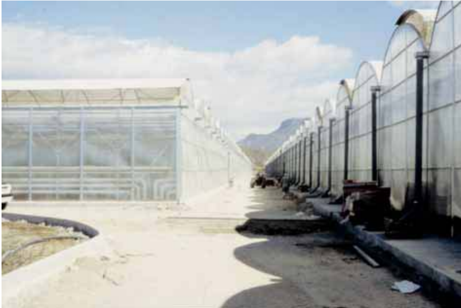
● : An example of the industrial greenhouses used in Spain (arc-shaped plastic multitennel). :.....
