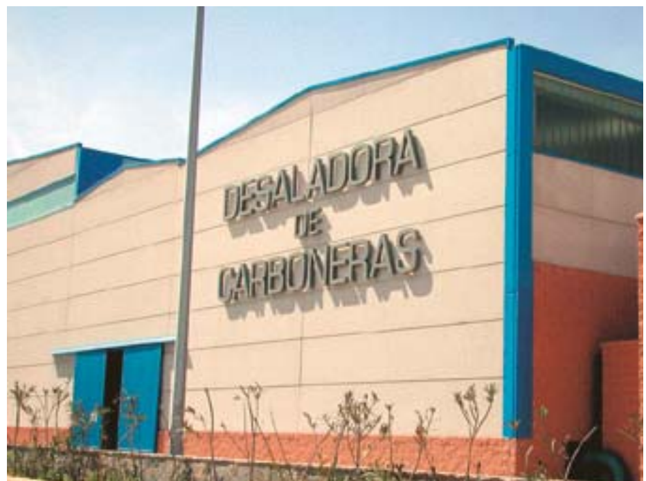
Figure 9. Seawater desalination plant in Carboneras, Almeria (Spain).
