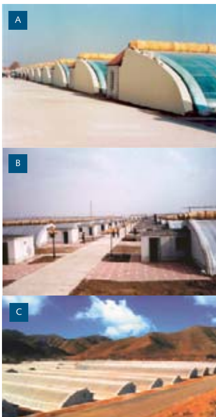
Figure 2. China's energy-saving greenhouse ranges. A. Note straw mat on ridges. B. A cluster of energy-saving greenhouses showing headhouses. C. Energy-saving greenhouse in mountainous area.
